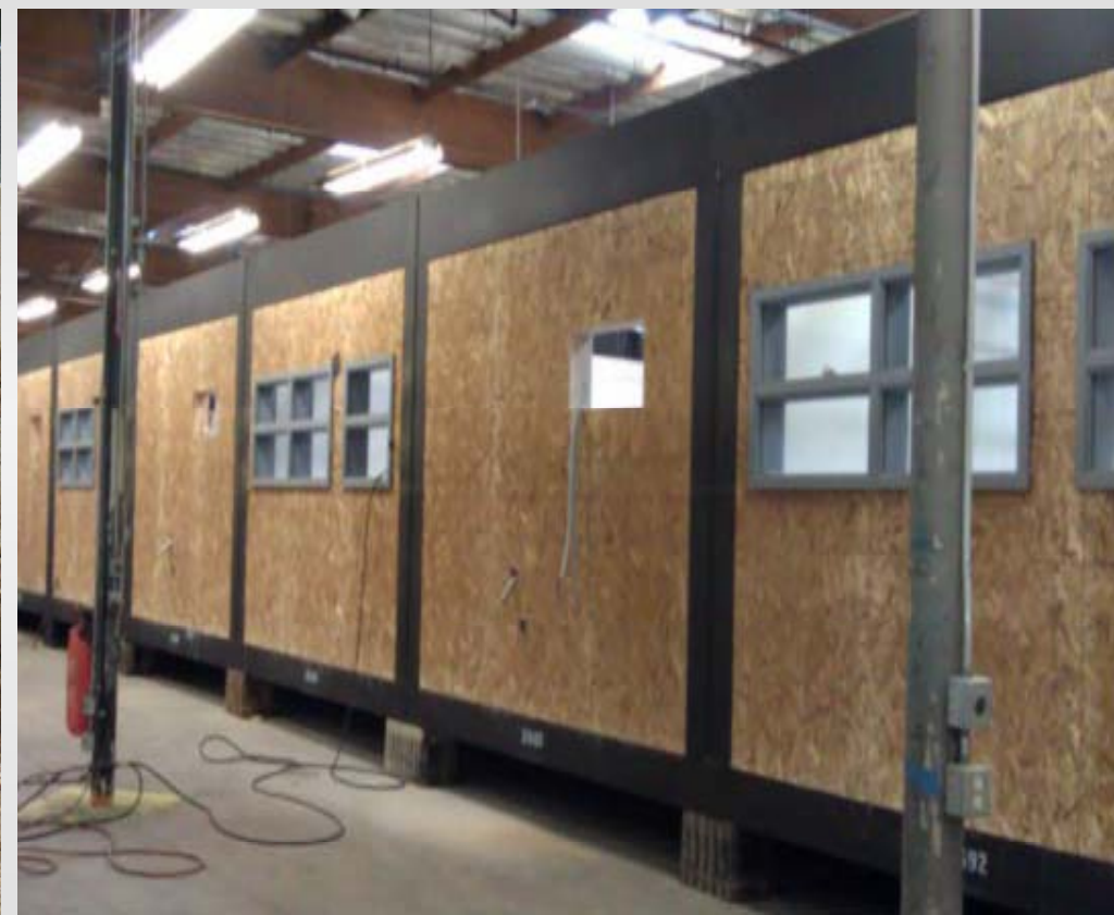
Building shell fabricated off-site
