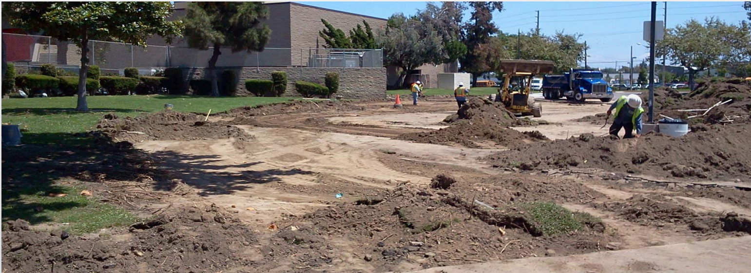
Parking lot improvements
